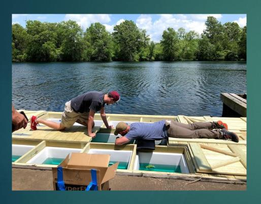
Unique design incorporates a basket/silo unit to allow easy access to seed and extend the oysters further into the water column, creating more water pressure and higher flow. Water from individual silos is discharged into a centrally located trough with a well and mounted pump to eliminate cavitation.
